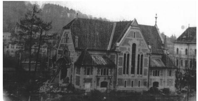
Figure 2. Picture during demolition
