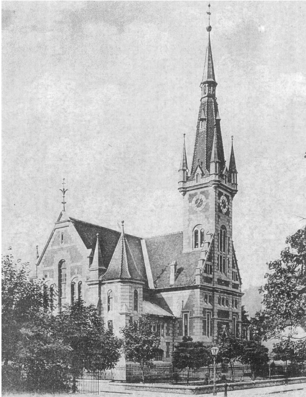
Figure 1. The Reformed church before demolition
